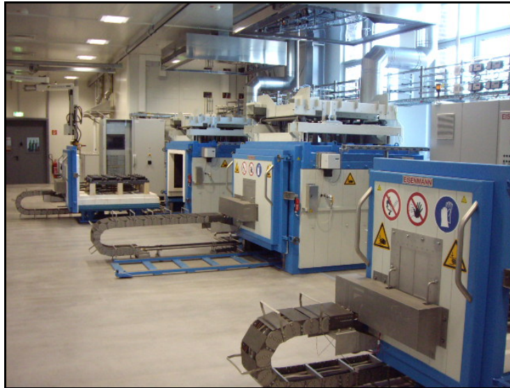
Figure 8 - Furnaces for Firing Fuel Cell Stacks
