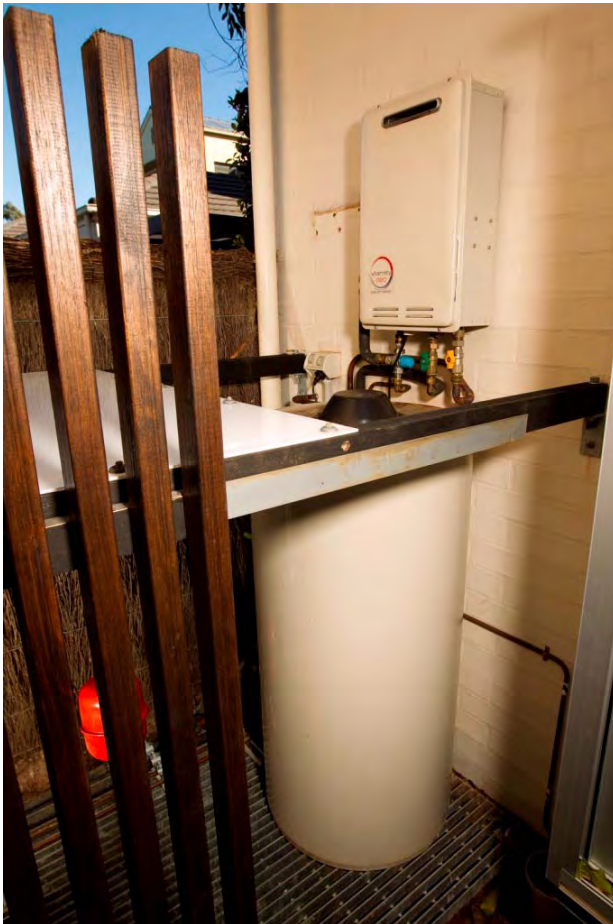
52 gal. hot water tank & booster
