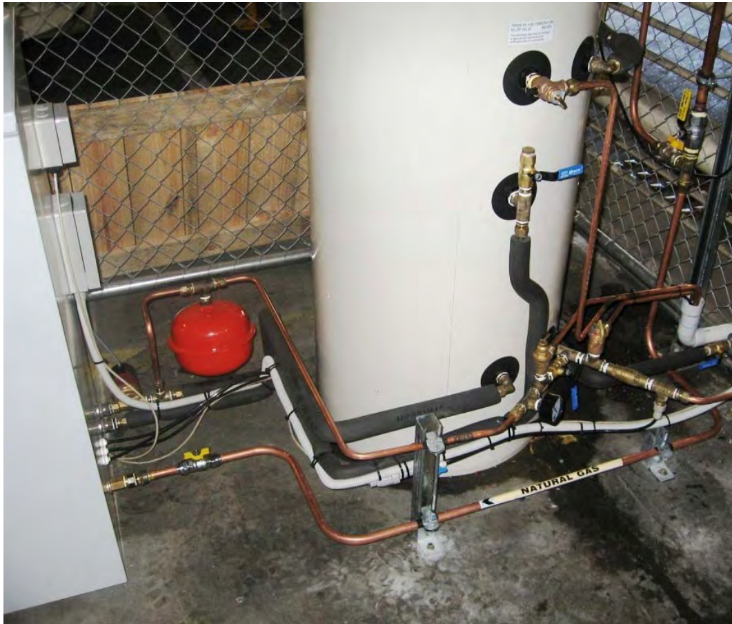
52 gal. tank thermal connections
